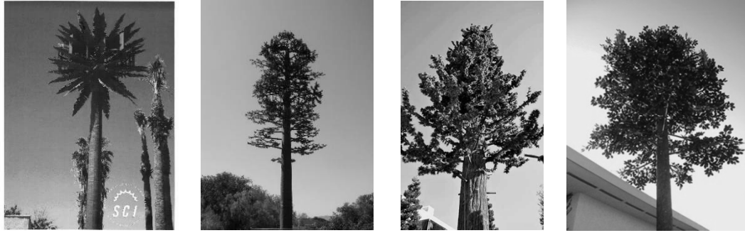
Examples of Faux Trees (Wireless Communication Facilities)
