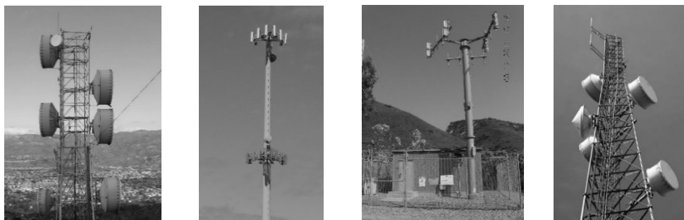
Examples of Non-Stealth Wireless Communication Facilities
