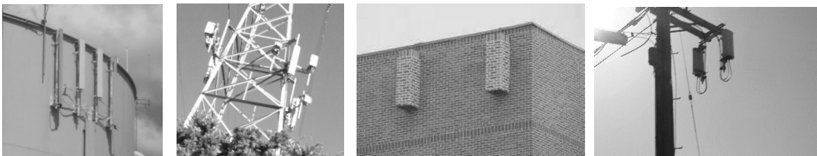
Examples of Flush Mounted Wireless Communication Facilities
