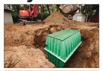
Since 2003, 116 AdvanTex Treatment Systems have been installed in Sunset Bay, a lakefront subdivision in northeast Tennessee, and 23 of these have been AX-RTs. According to Arthur Helms, Helms Construction, the RT's are "a lot easier to install. This one only has a few connections, so you can't hardly screw it up." Even better, Helms says that the RT "saves about 8 hours labor and saves on fittings ... I make more money with the RT. I can do it and go on to the next one."
