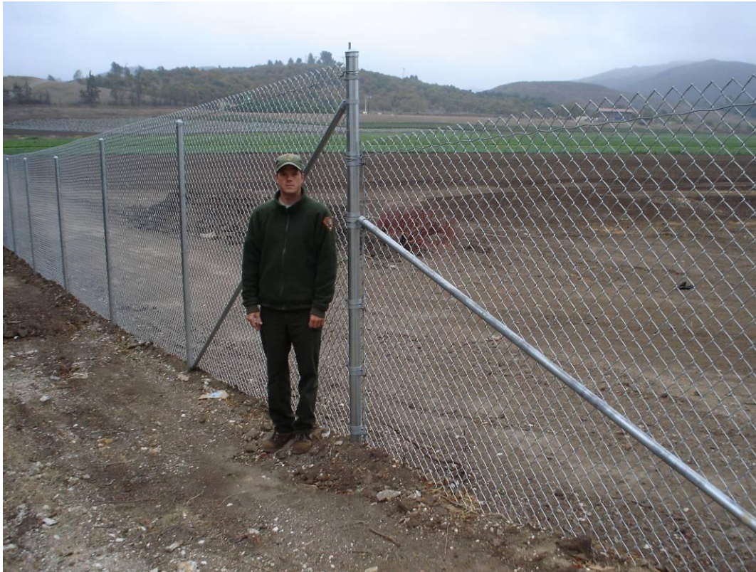
Figure 3. Chain-link wildlife exclusion fence buried 2 feet into the ground with a total height above ground of 6 or 8 feet.
