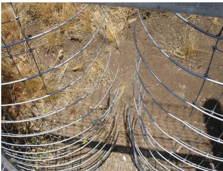
Figure 6. Gap between tine ends to allow flexing at the point an animal would pass through.
