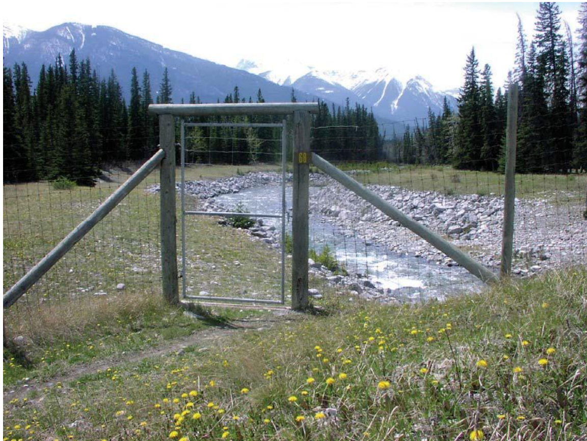
Figure 29. Spring-loaded swing gate in wildlife exclusion fence (Credit: Tony Clevenger).
