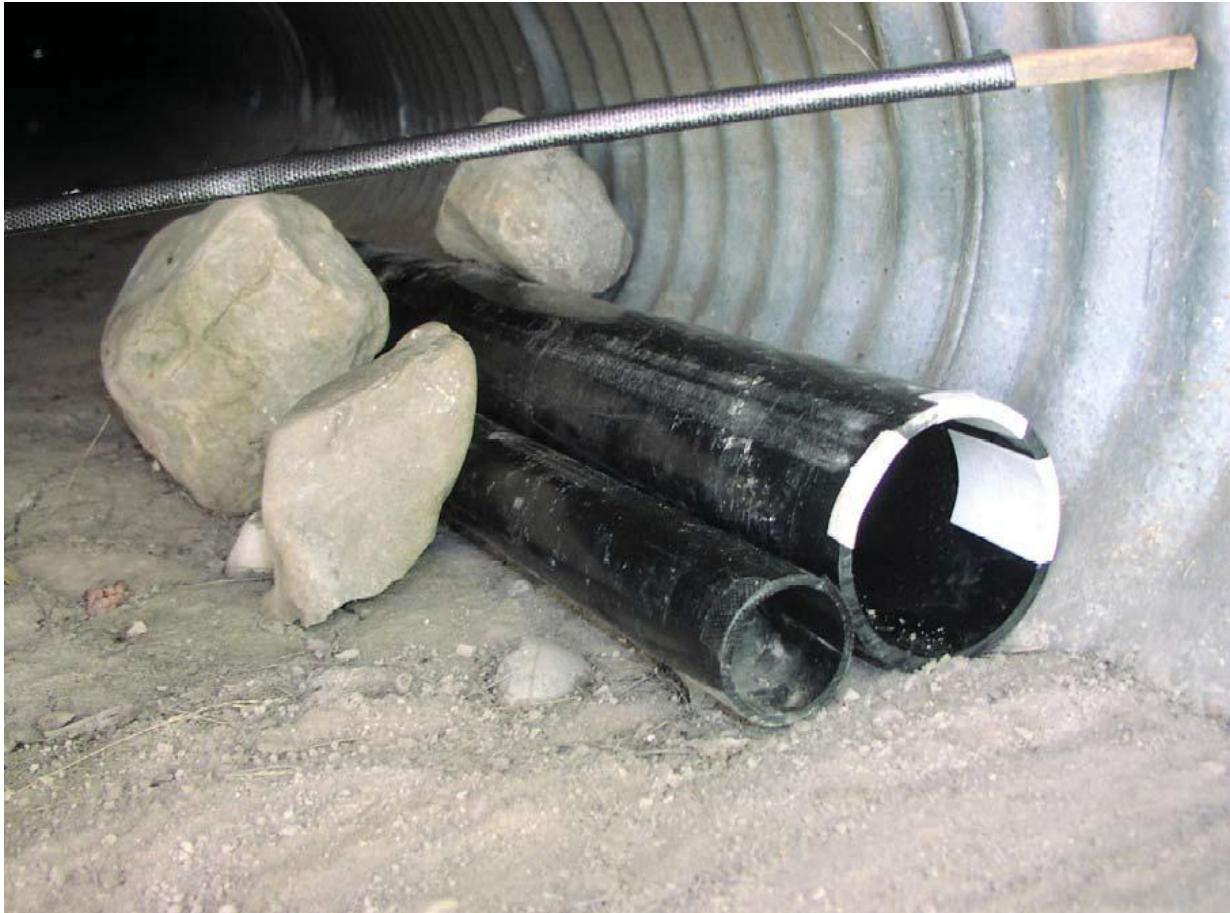
Figure 32. Example of pipes placed in culvert to provide cover for small mammal passage (Credit: Tony Clevenger).
