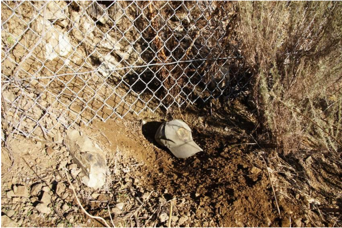
Figure 23. 23cm gap under the wildlife exclusion fence. Tracks of coyote and raccoon have been found at this location going under the fence and accessing the right-of-way.
