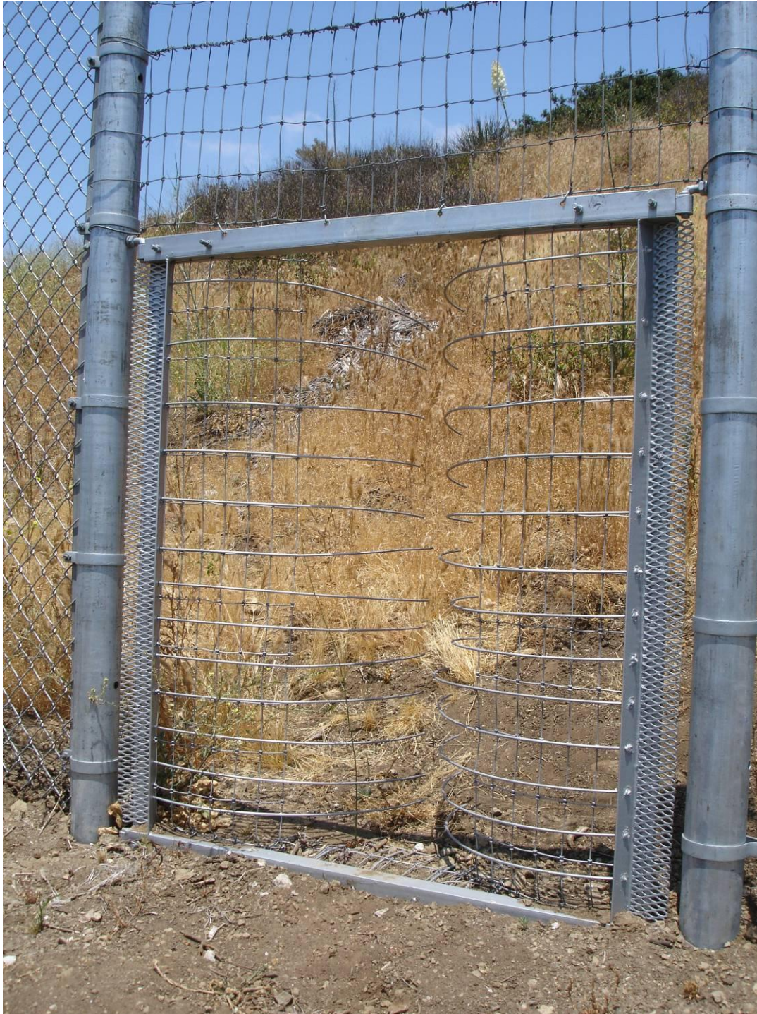
Figure 4. One-way gate designed to allow animals that are trapped inside the right-of-way to safely exit.
