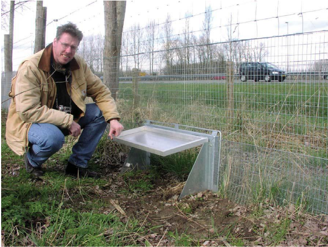
Figure 31. Small hinged door in wildlife exclusion fence for escape of medium-sized mammals (Credit: Tony Clevenger).
