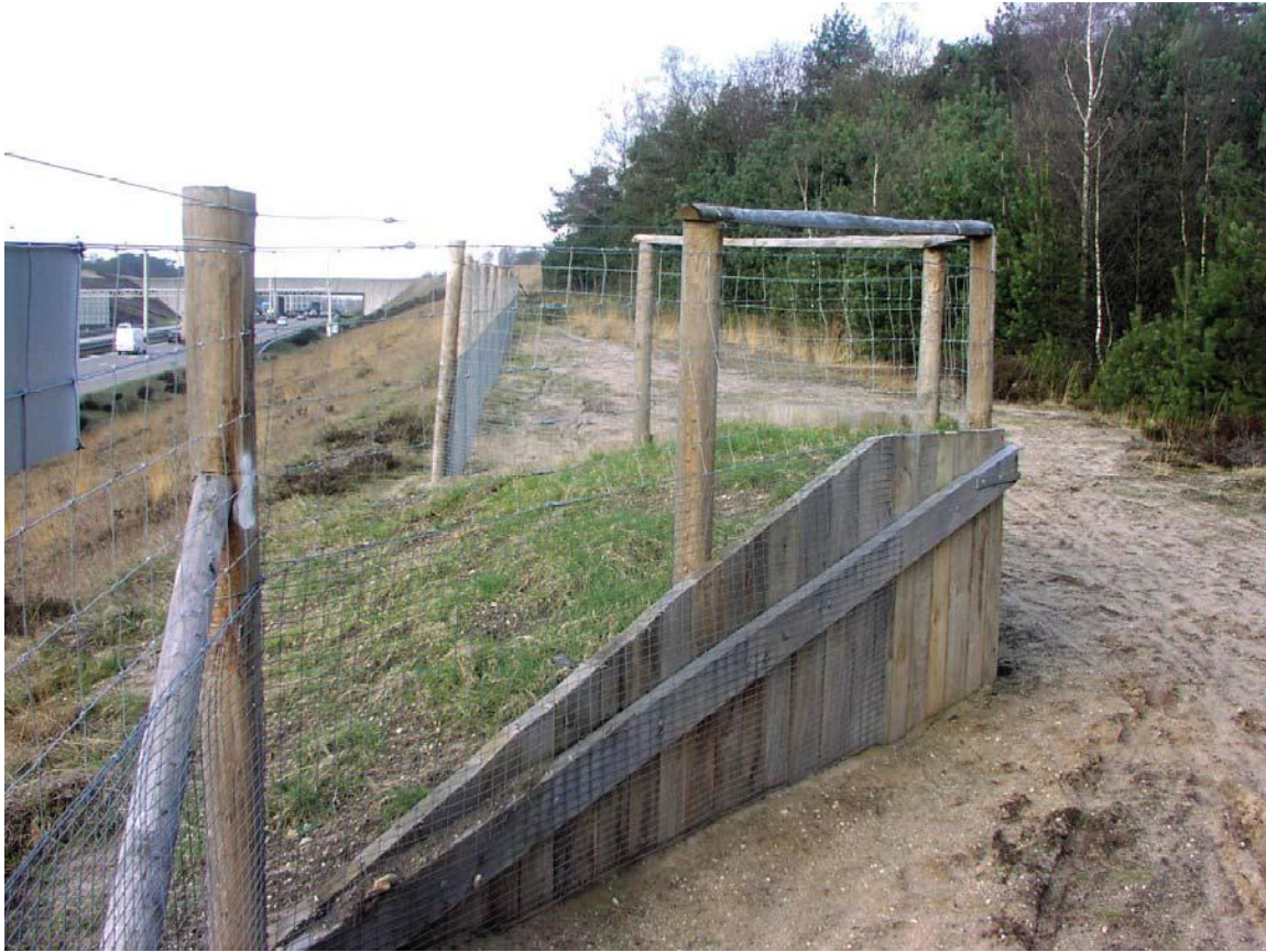
Figure 30. Examples of escape ramp (jump-out) for wildlife trapped inside the fenced highway right-of-way (Credit: Tony Clevenger).
