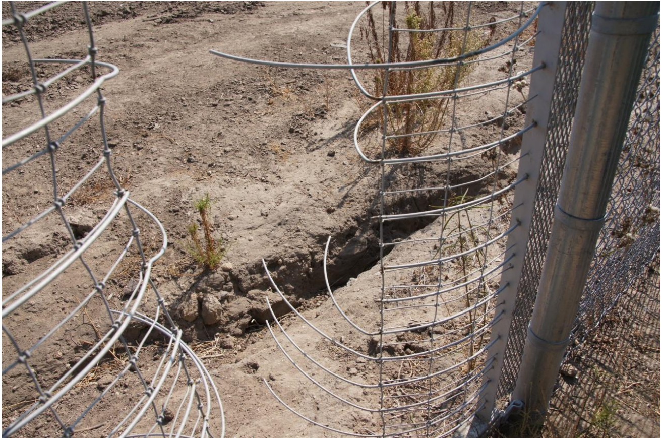
Figure 27. Tines bent and broken off from people using the one-way gate.
