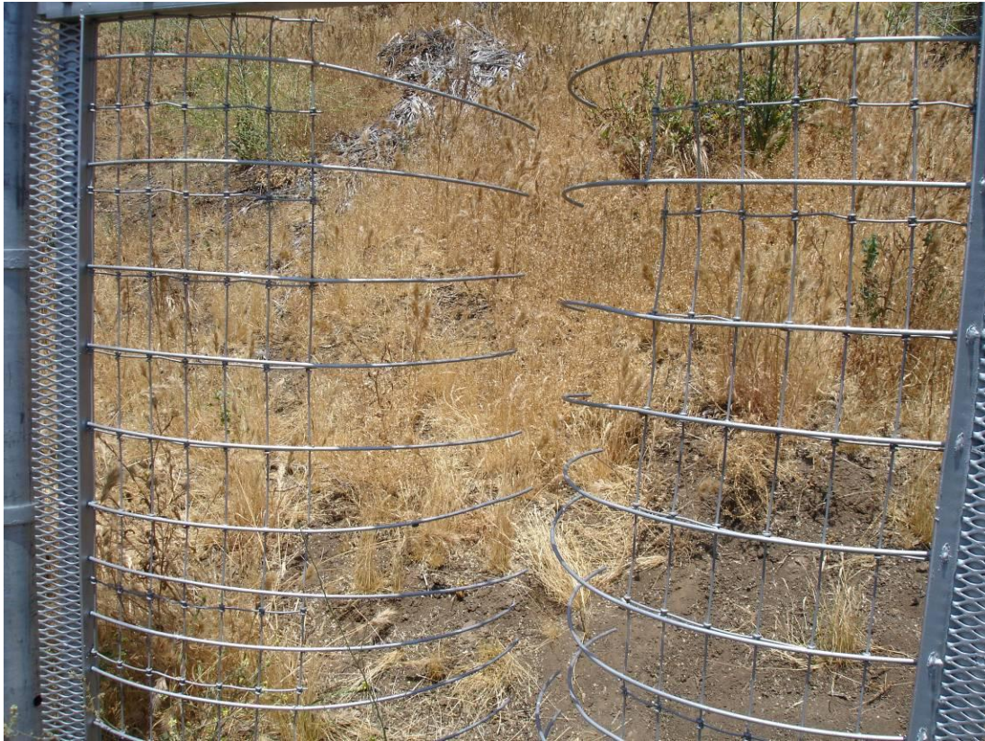
Figure 5. Wire mesh secured on the one-way gate tines to prevent flexibility that may allow animals to bend the tines and squeeze through.
