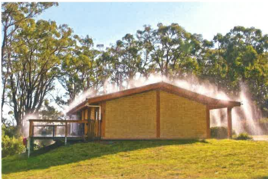
Figure 7. Exterior Sprinklers. As a wildfire approaches, exterior sprinklers wet the structure at risk, the surrounding environment, and increase humidity to prevent ignition. Photo: Platypus Fire Pty Ltd.
