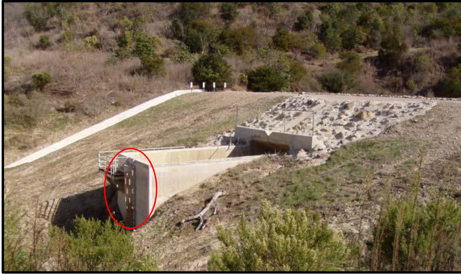
Figure 3-1 This debris basin includes a perforated “debris bleeder” made from a corrugated metal pipe (circled in red). (Source: VC Watershed Protection District)
