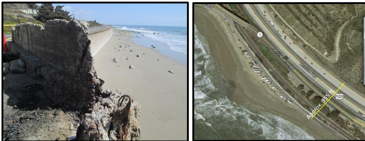
Figure 2-4. A damaged seawall at Emma Wood State Beach protects a thin stretch of shoreline that includes the State Park access road, the rail line, Old Coast Highway, Highway 101, and power, oil, gas, and sewer lines. The bottleneck of infrastructure on a thin stretch of the shoreline is shown in the Google Earth image below.
