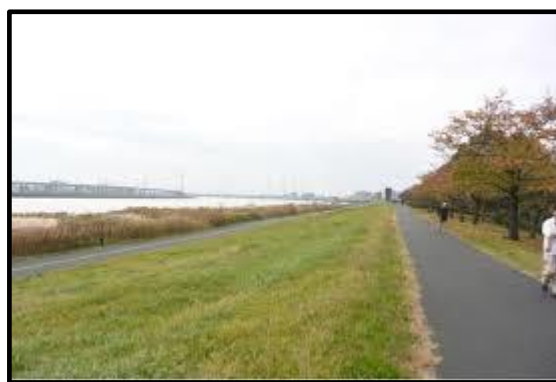
Photo 3-6: This horizontal levee provides a transition area between an estuary and an orchard that includes recreational pathways.
