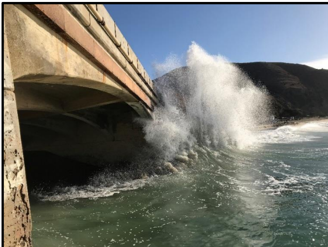
Photo 3-1: Sycamore Canyon Bridge located on the South Coast is 80+ years old and needs to be replaced. The new bridge will be built at a higher elevation.
