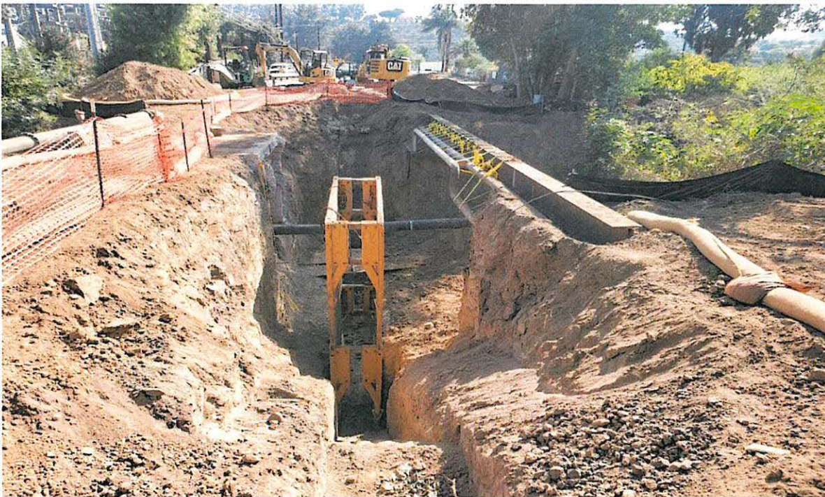
Excavation with 1:1 Slope at Project Site
