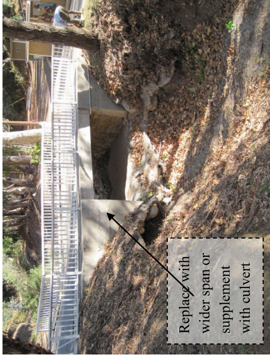
Road bridge #2 is undersized for the channel and flows resulting in channel incision and flooding.
