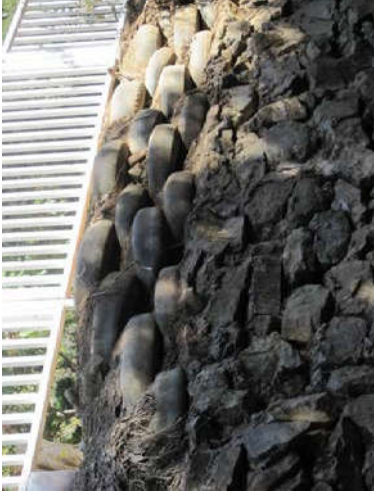
Close up of tire bank stabilization
