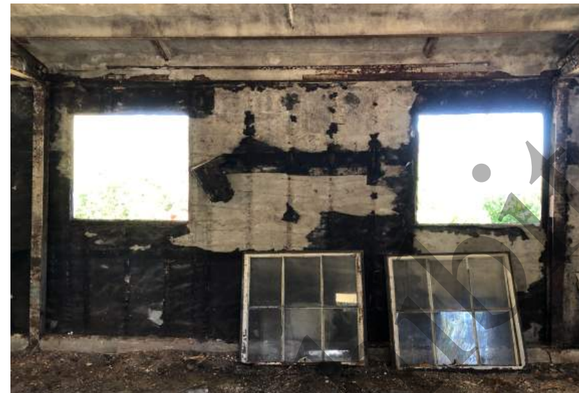
Studs and water membrane gone
