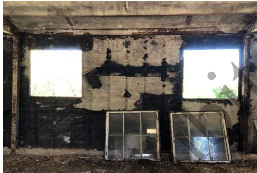
Studs and water membrane gone
