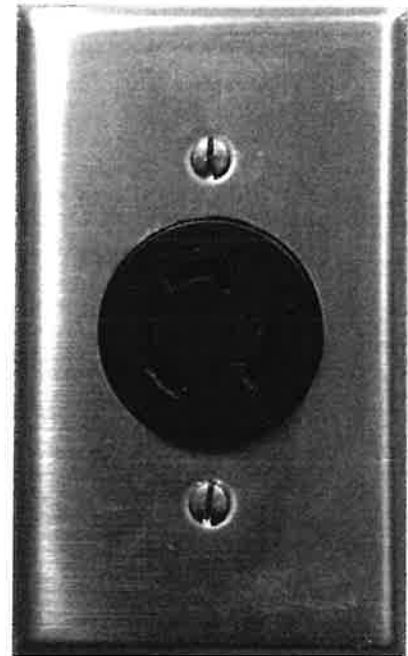
Example of L6-20 Twist-Lock Outlet
