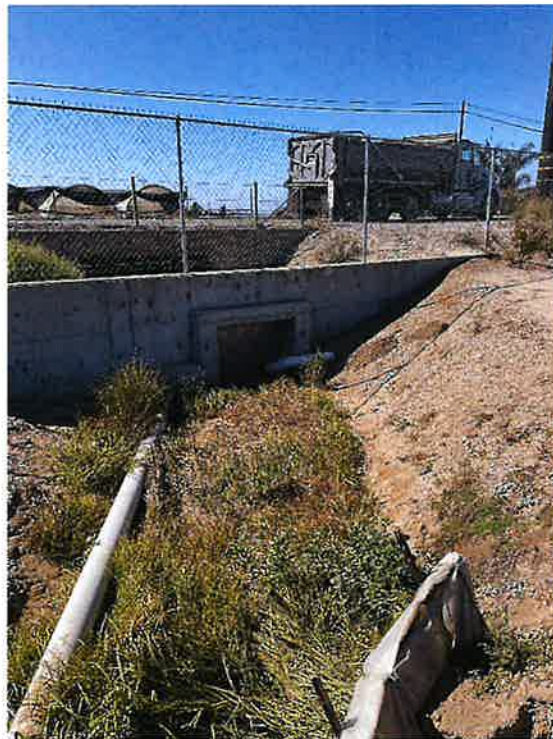
Figure 3: Flood Wall with Flap Gates (along State Route 118)
