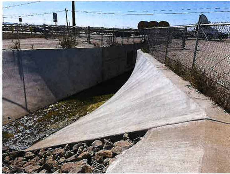
Figure 2: Concrete Transition and Box Conduit (downstream end of Ferro Channel at State Route 118)
