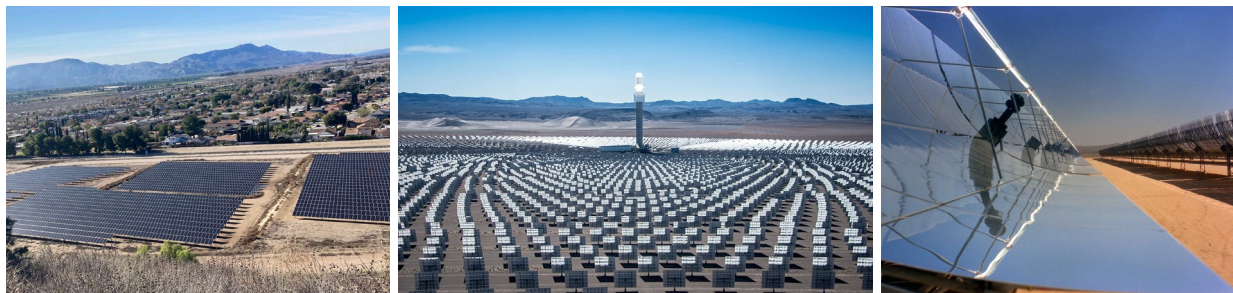
Figure 1: Types of Solar Arrays - PV (Left), Solar Tower Concentrator (Center), and Solar Line Concentrator (Right)
